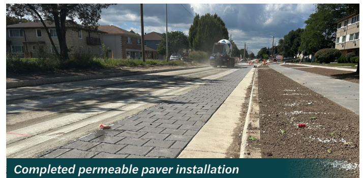
Permeable paver installation operations
