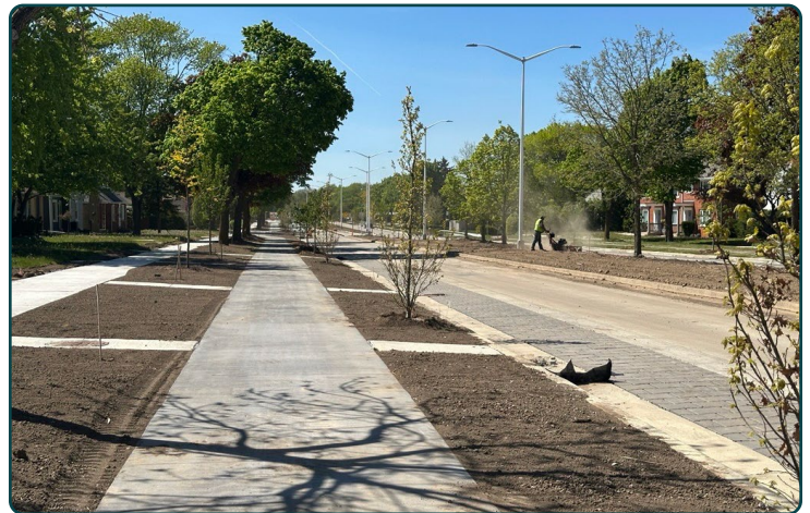
Landscape Restoration in Reconstructed Eastbound Lane
