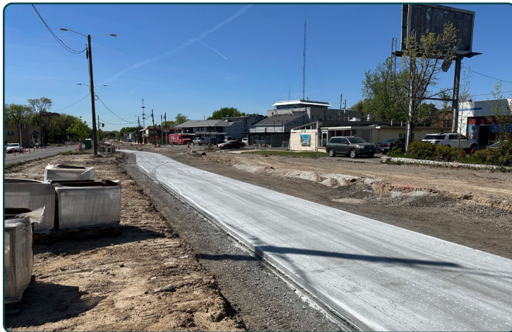
Paving Operations on W. Lisbon Avenue
