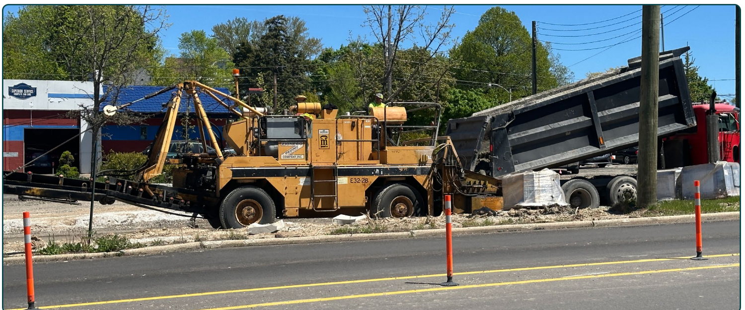
Paving Operations on W. Lisbon Avenue
