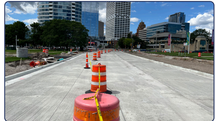
Both travel lanes poured on E. Michigan Street from LMD to AMD
