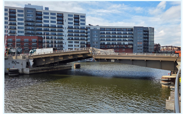
Water Street Bridge painting operations nearly complete
