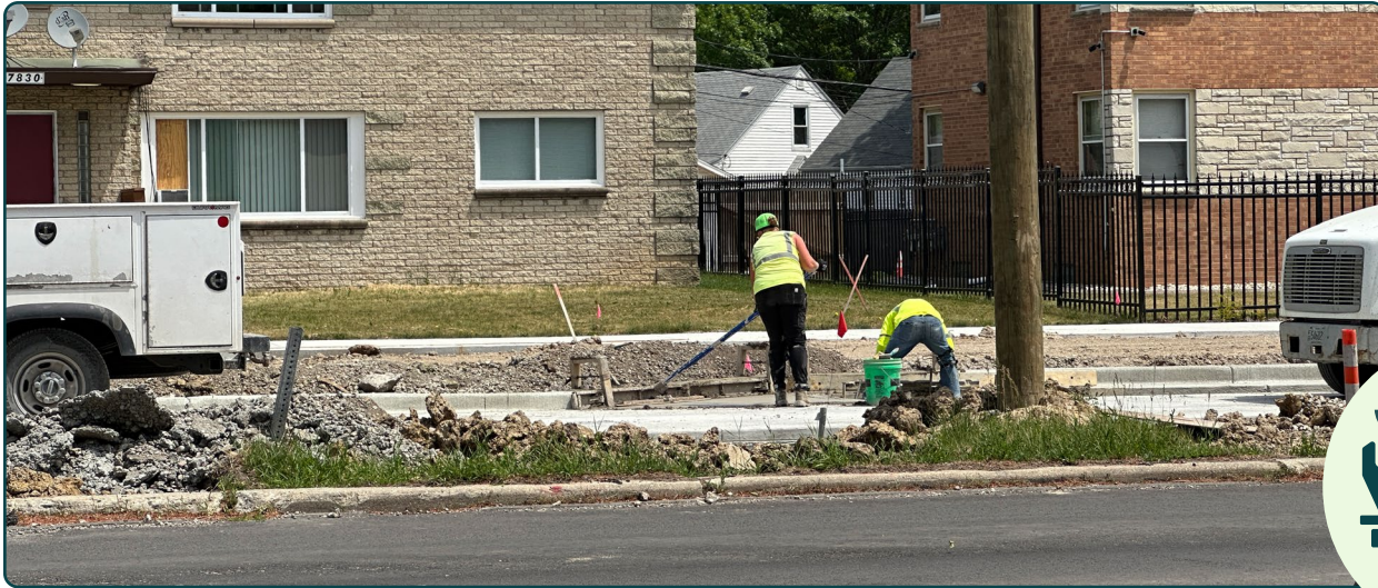
Hand-pouring concrete on W. Lisbon Avenue.
