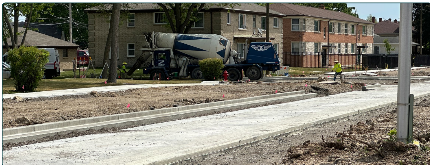
Hand-pouring concrete on W. Lisbon Avenue.
