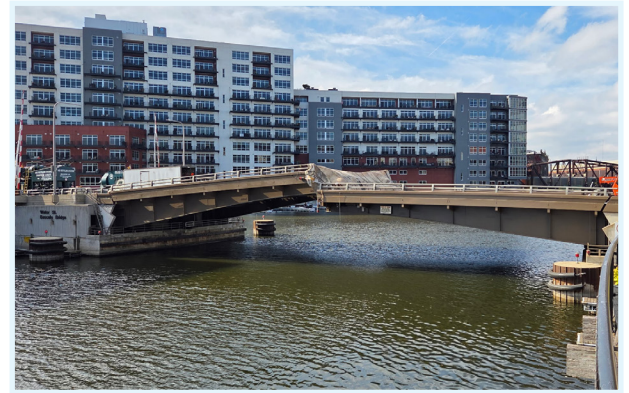
Water Street Bridge painting operations nearly complete
