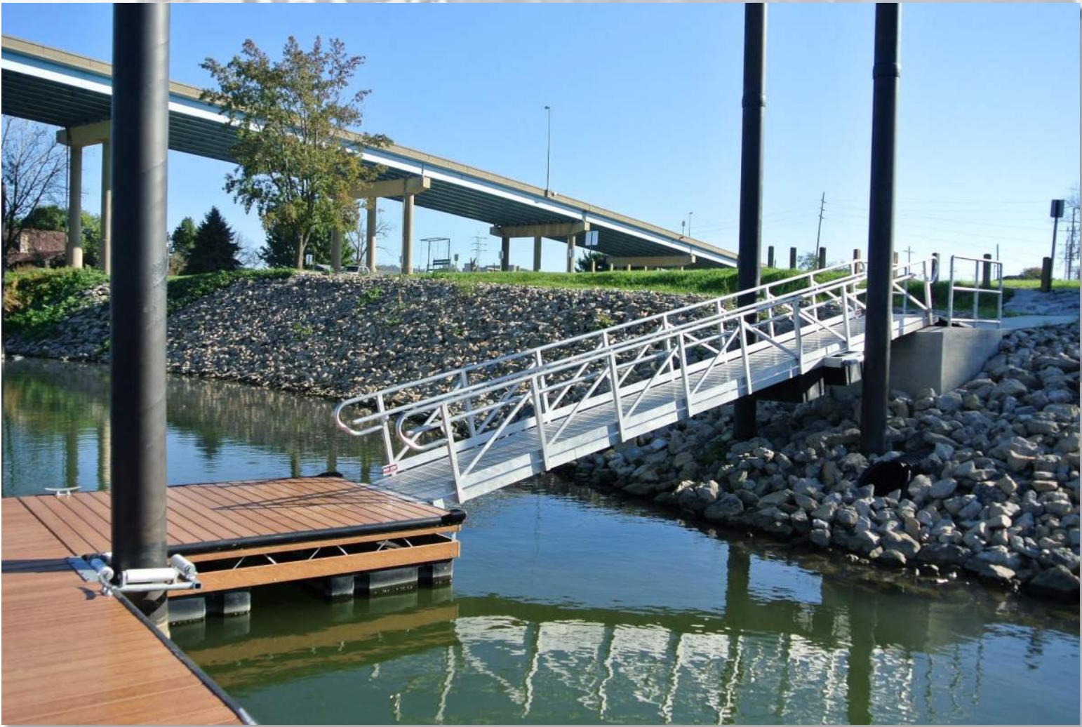
NEGOTIATING 12 FEET OF VERTICAL CHANGE FROM THE RIVERWALK TO THE RIVER REQUIRES MULTIPLE GANGWAYS TO FACILITATE UNIVERSAL ACCESSIBILITY.
