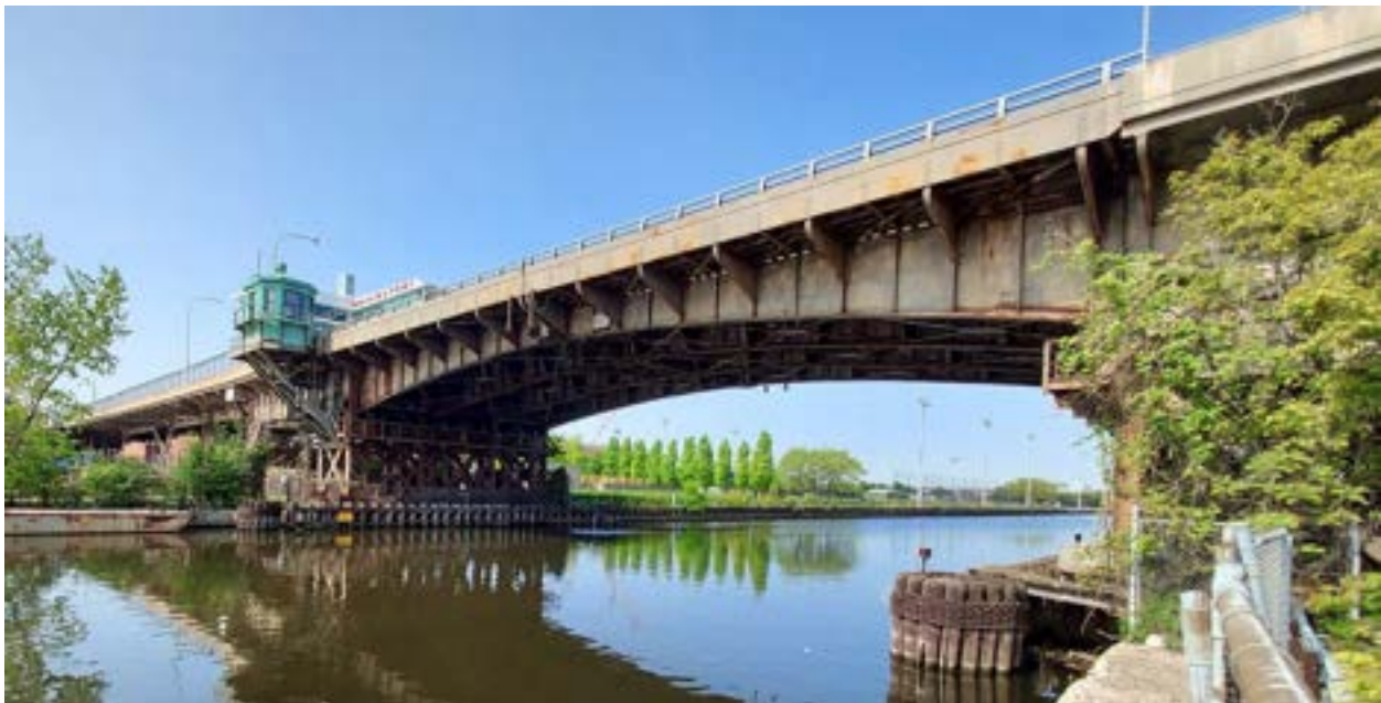
FIGURE 1: Existing bascule span over the Menomonee River. View looking southwest from north bank. June 2023.
