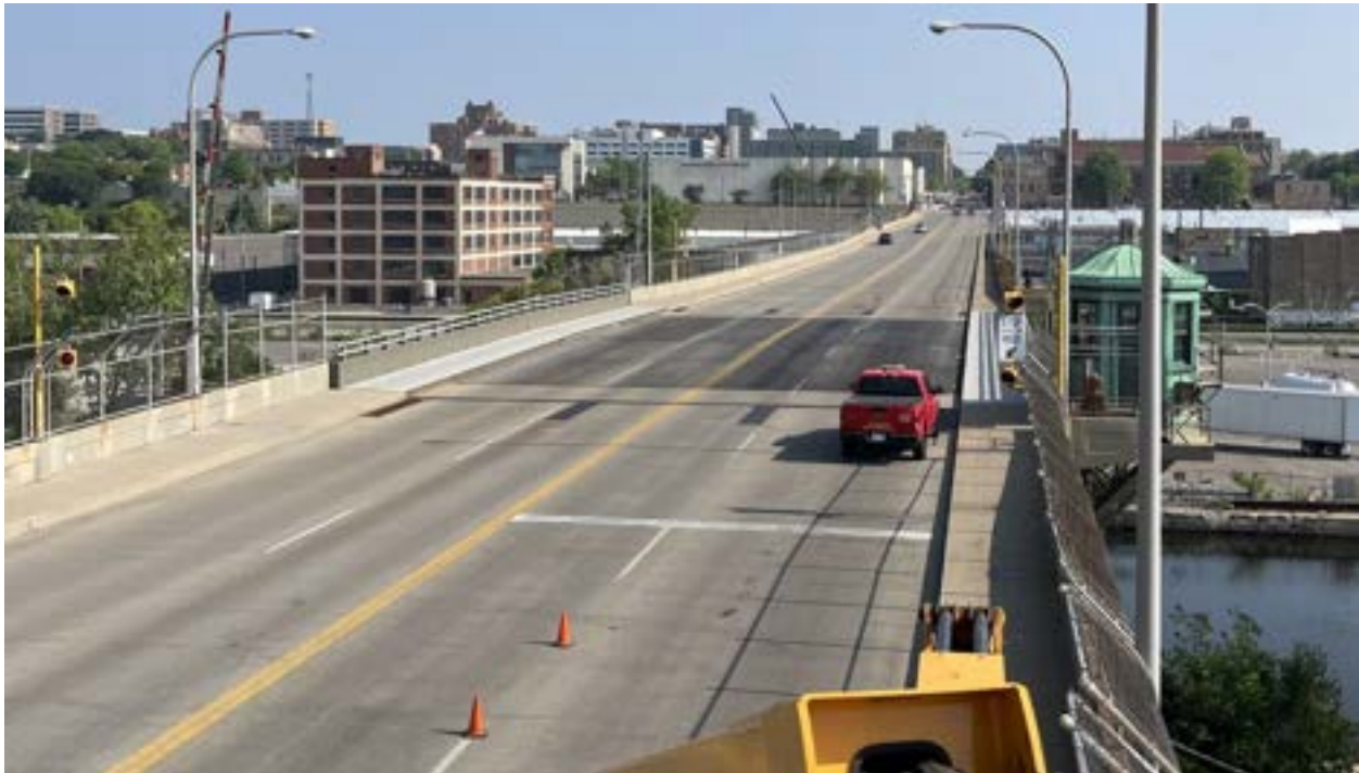
FIGURE 2: Unit 14 bascule span and approach spans of the 16th Street Viaduct looking north. June 2023.
