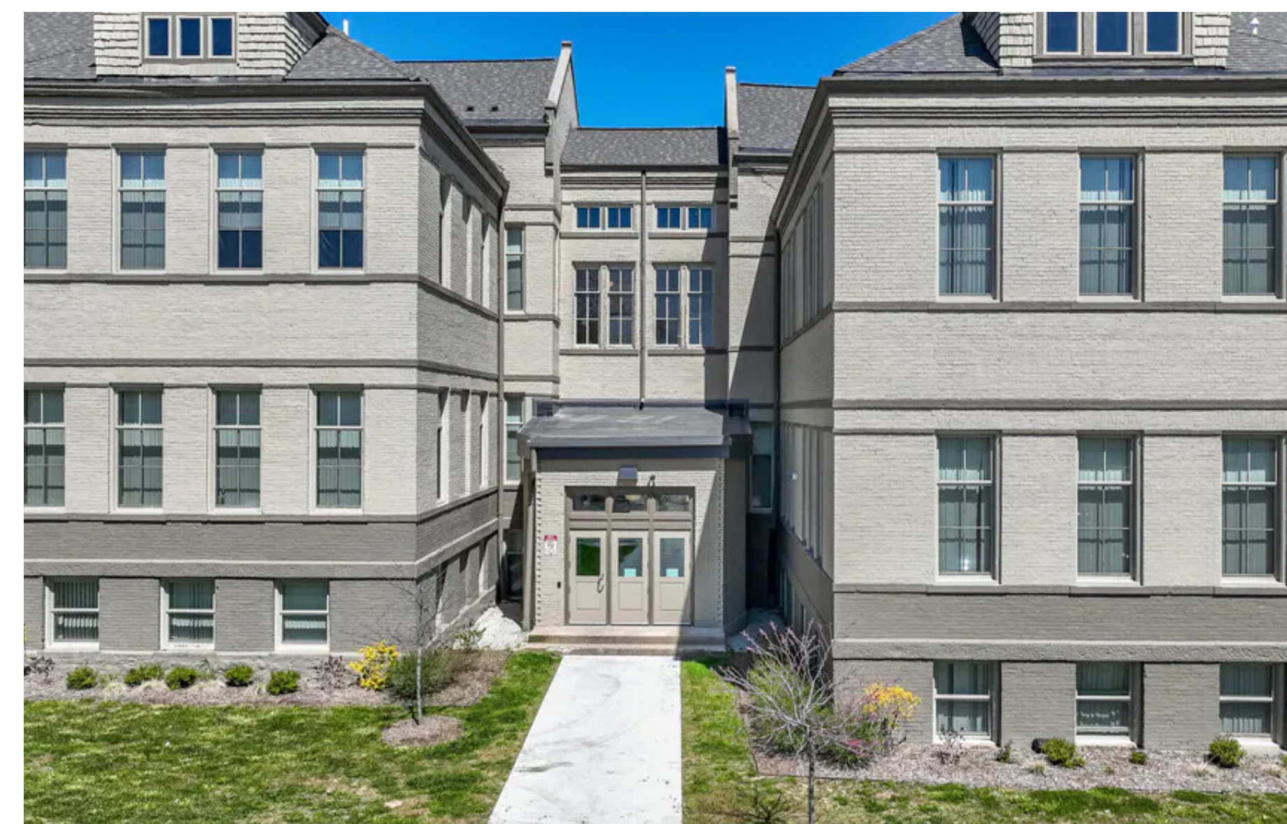
Example of adaptive school reuse
