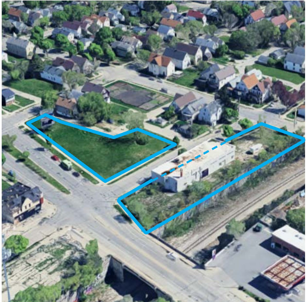
Image 94. Aerial image of the Site 5 properties.
