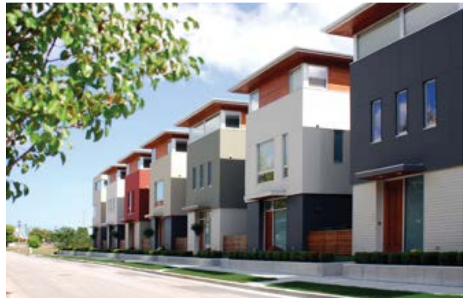
Image 18. Front doors to townhomes
