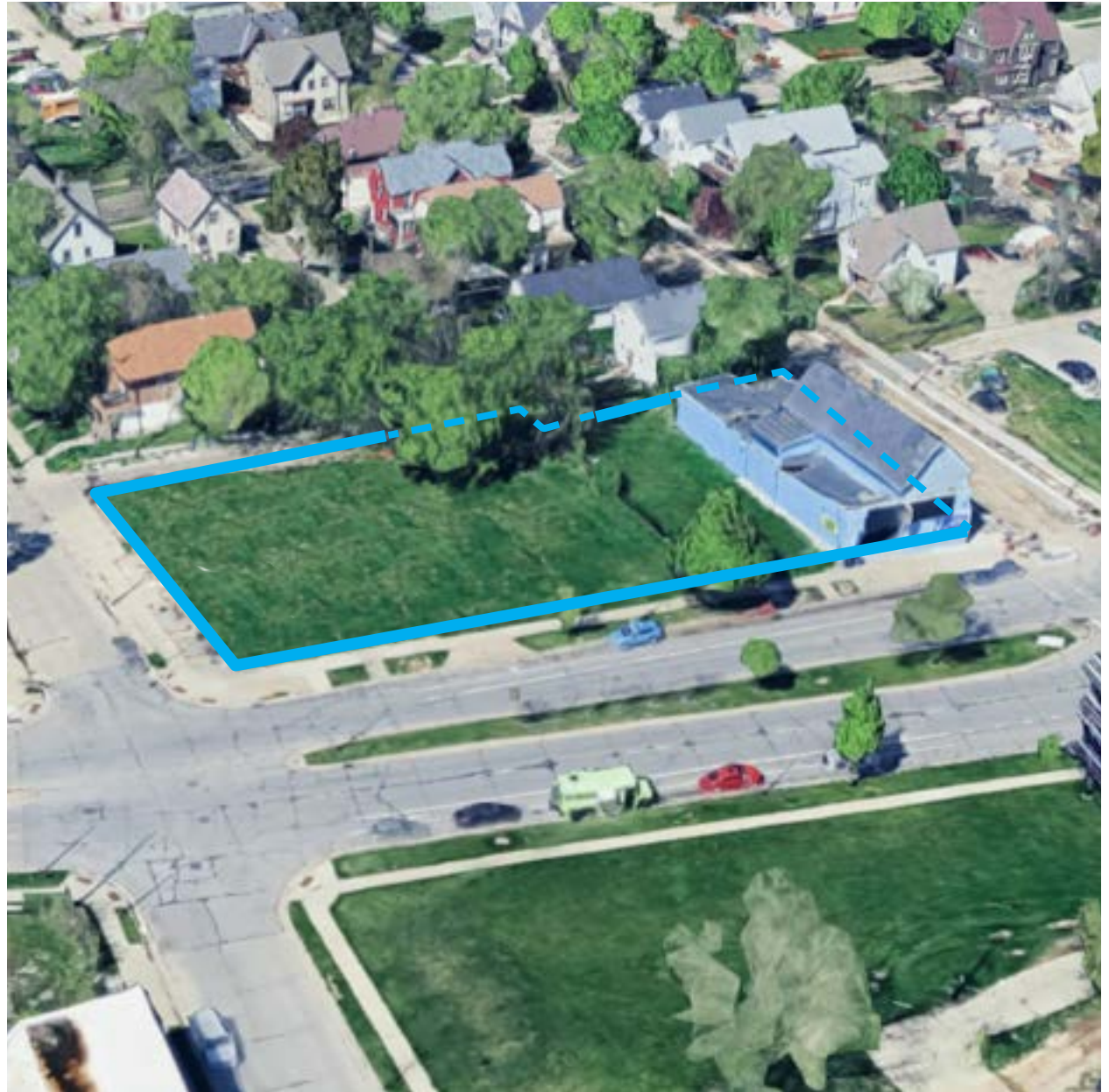
Image 102. Aerial image of the Site 6 properties.
