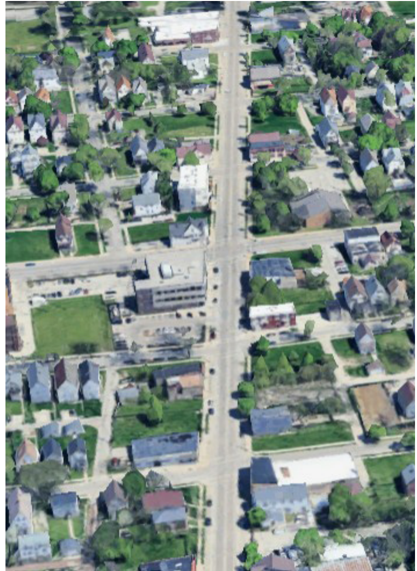
Image 2. Aerial photograph of W Lisbon Avenue
