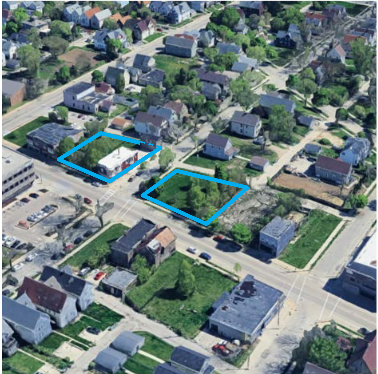
Image 61. Aerial image of the Site 2 properties.
