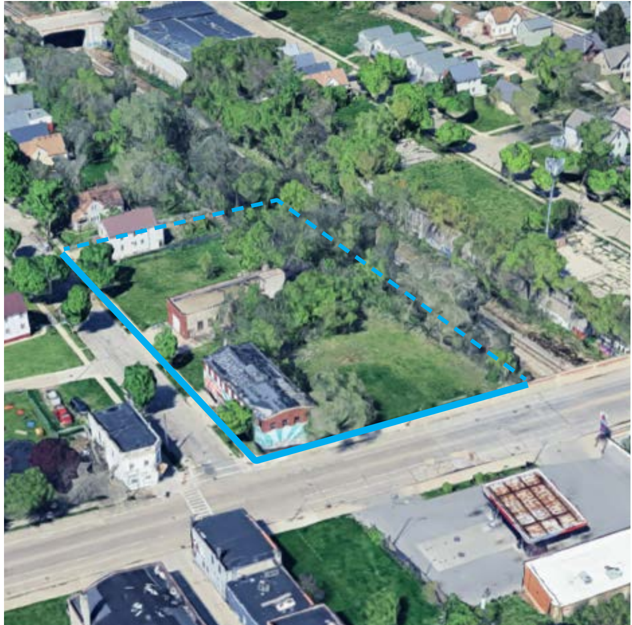
Image 84. Aerial image of the Site 4 properties.
