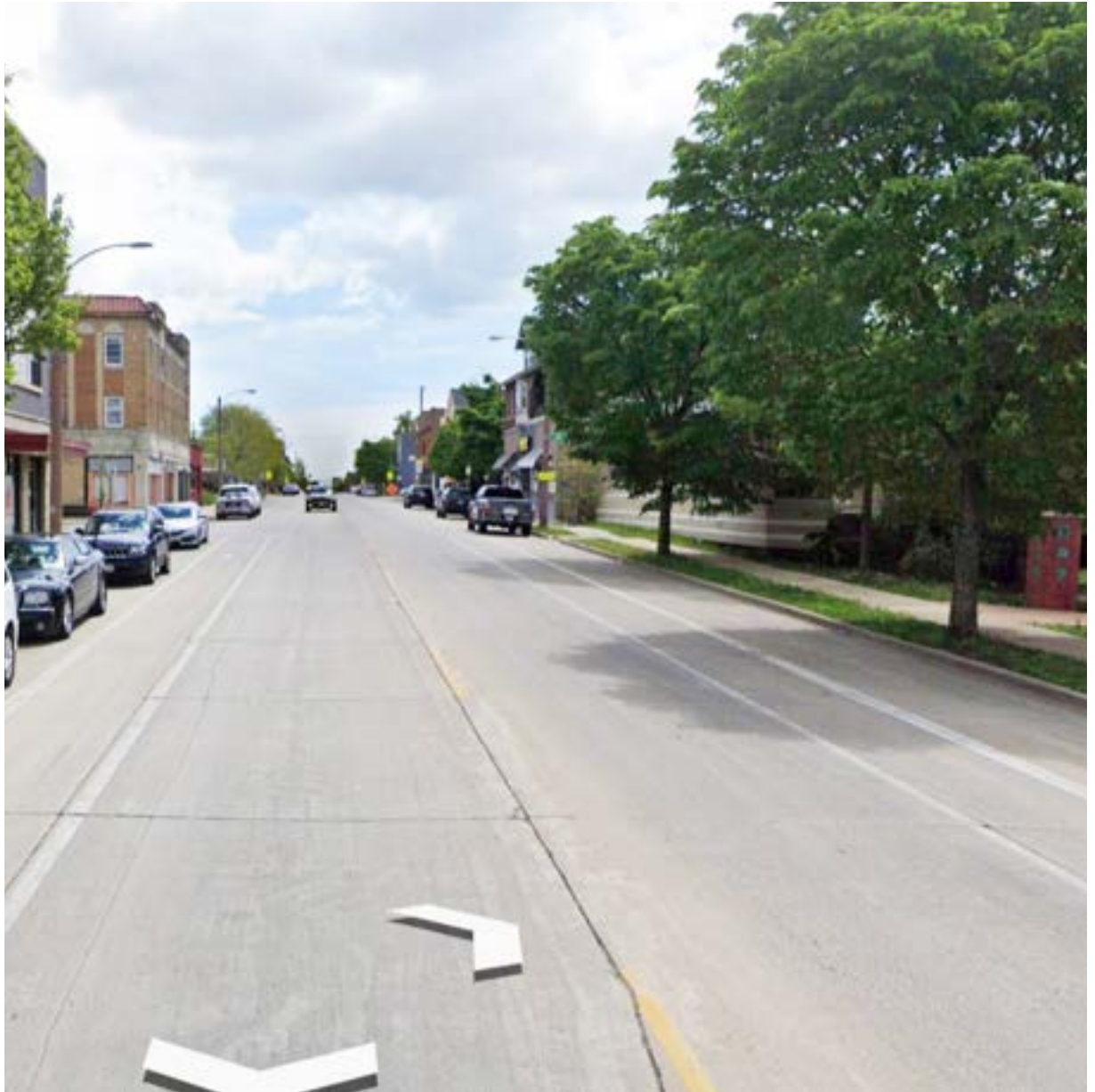
Image 10. Current condition of the Walnut-Lisbon Avenue corridor.
