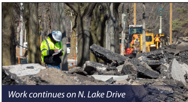
Pavement removal on N. Lake Drive
