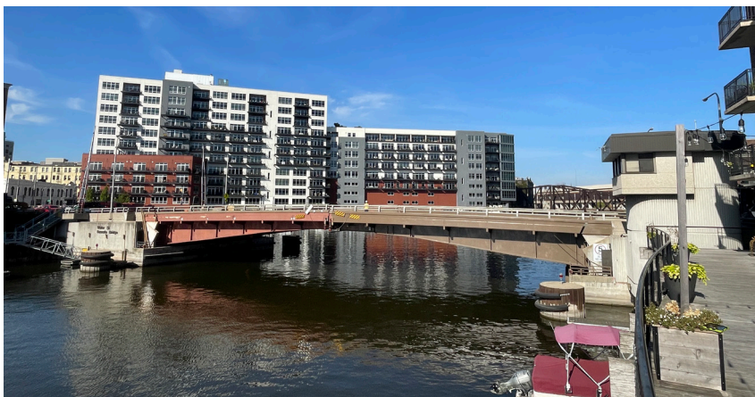
North bascule span painting complete
