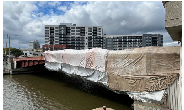
North bascule span painting in progress
