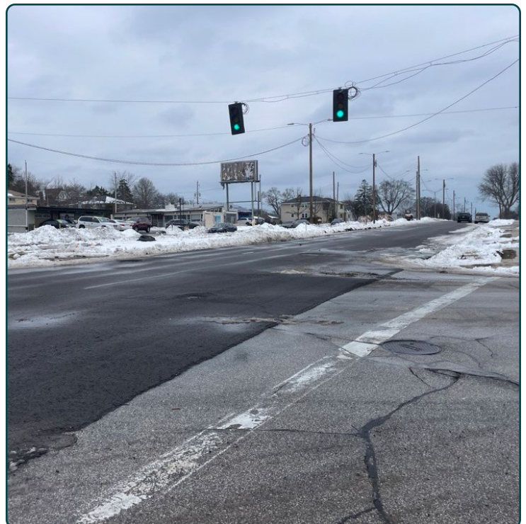
Temporary Asphalt on Lisbon Avenue.
