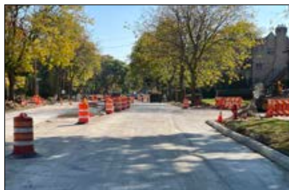
New pavement on N. Lake Drive near E. Kenwood Boulevard
