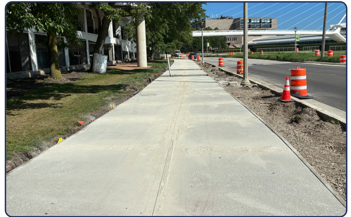
Sidewalk poured on the west side of N. Lincoln Memorial Drive
