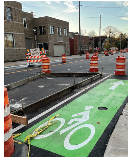
Pinned-on concrete island form next to freshly painted bike lane
