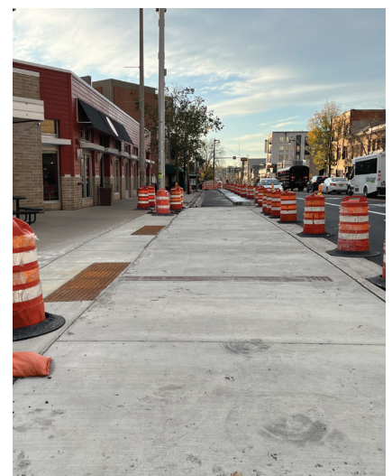
Concrete bus boarding island; green bike lane paint to be installed next spring
