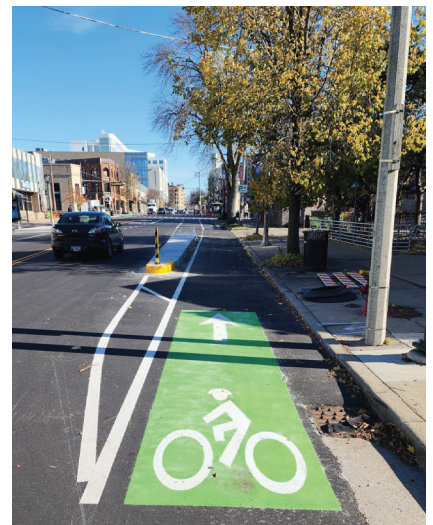
High visibility bike lane pavement markings
