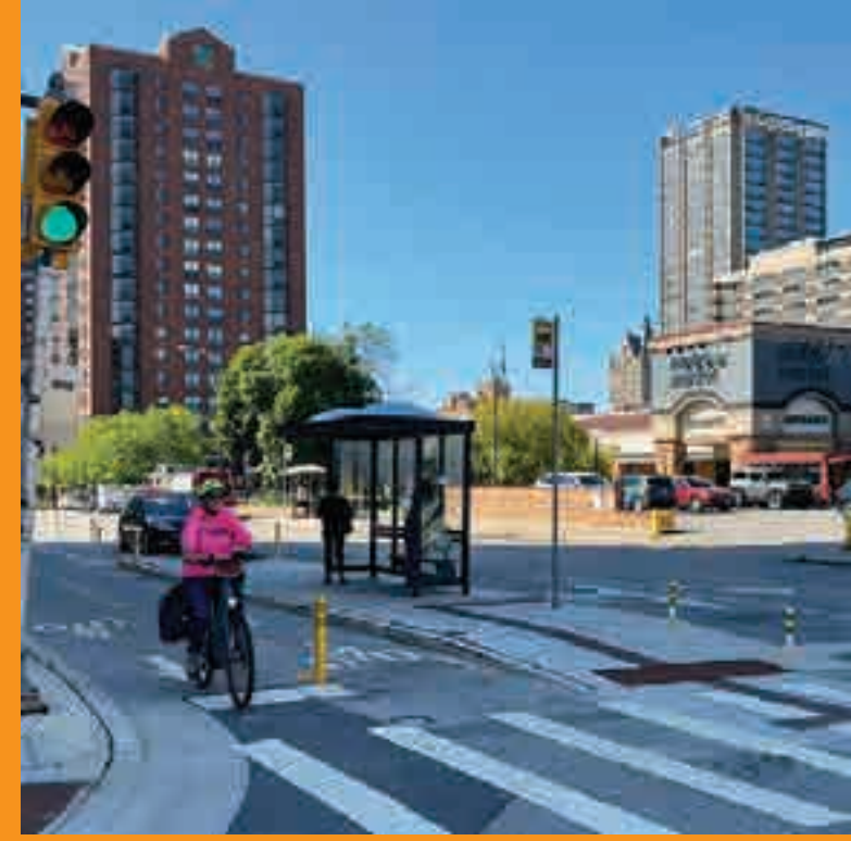
Protected Bike Lane
