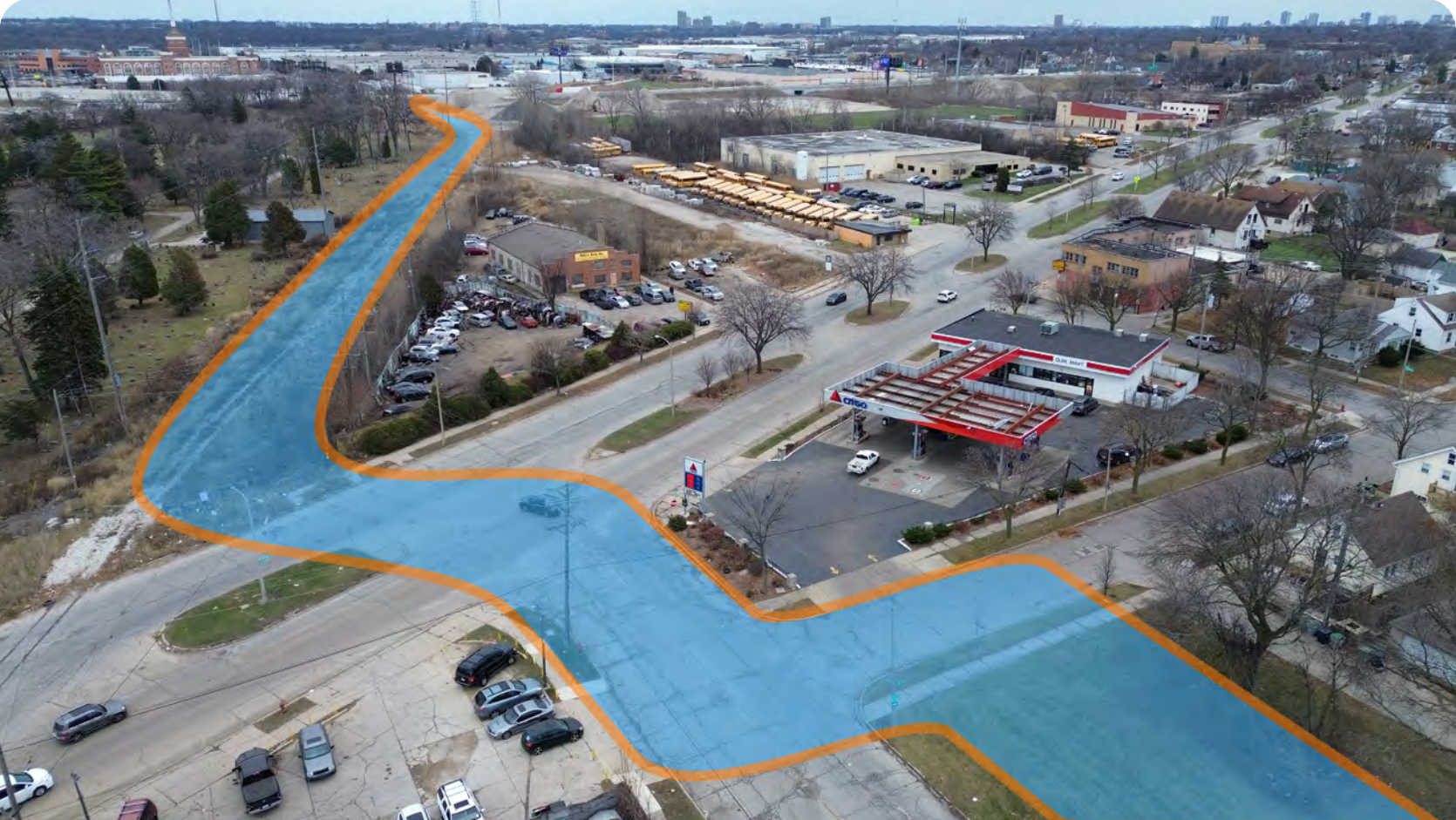
Beerline Trail Crossing at Green Bay Ave
