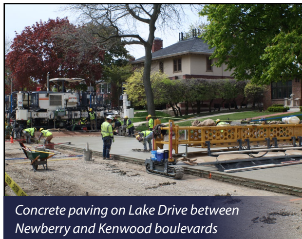
Concrete paving on Lake Drive between Newberry and Kenwood boulevards
