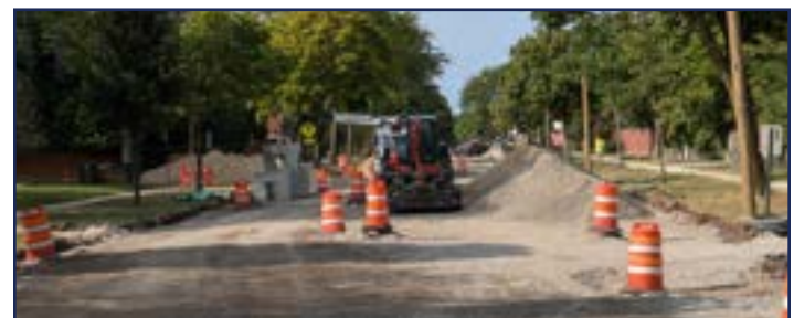
Over the last two weeks crews worked on replacement of underground utilities
