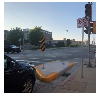
Concrete Bump Out
