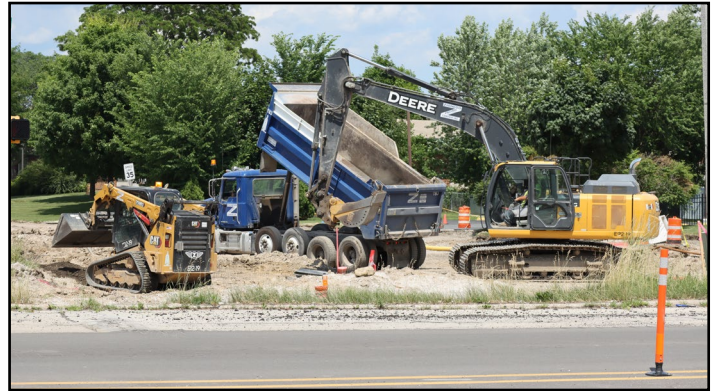
Pavement removal operations | July 2025
